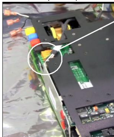
Step 10 Inspect the AC power connector
